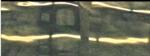
Polished concrete surface is dependent on the concrete floor flatness. Less flat the concrete, more waviness concrete will appear
