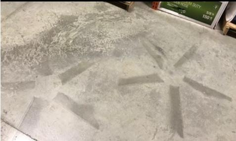
Be careful NOT to leave equipment, boxes, tape, etc. on the concrete... IT WILL PRODUCE A SHADOW.
